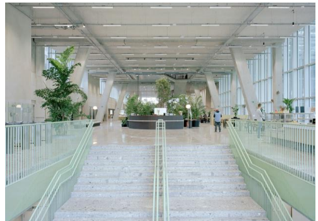
Figure 12 View from level 1 - deviation structures
