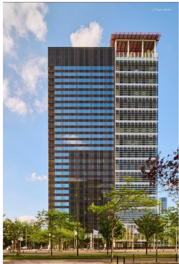
Figure 15 a/b : ZIN after construction
