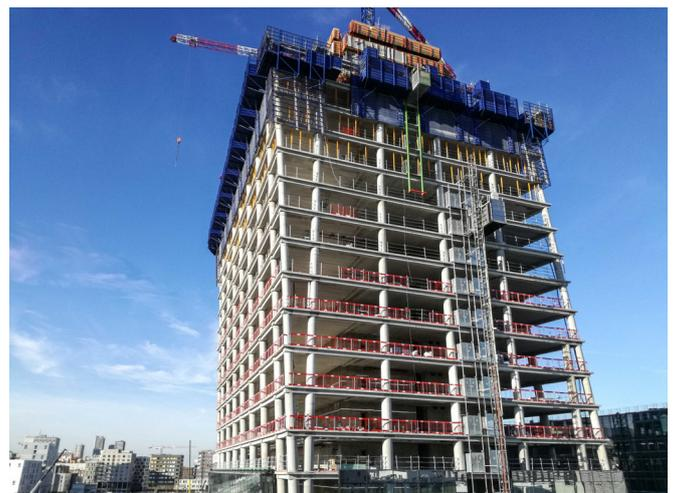
As the façade columns are inclined, the side thrust forces must pass through the structure to be transmitted to the core. In addition, particular attention was paid to checking compliance with standards in terms of acoustic criteria and fire resistance.
