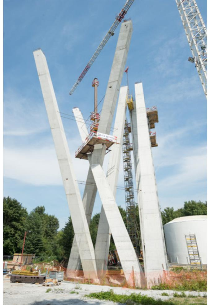
The water tower is built to store 2,000 m<sup>3</sup> of water 40 m above the ground.
