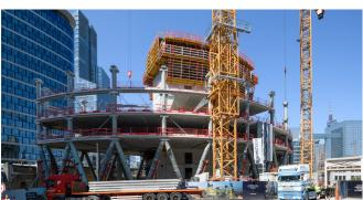
Office tower with a global surface aera of nearly 53 500 m² consisting of seven underground levels (+/- 10 000 m²) for parking of 168 cars and archive rooms, a ground floor and thirty-three office levels (+/- 43 500 m²). On a narrow site, surrounded by public spaces and railway lines, the geometry of the building is characterised by an elliptical lens 28 m wide and 69 m long. With a height of 128 m high (137 m including the façade structure), it qualifies as a high-rise building.
