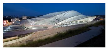
The new station is composed of a monumental 200-meter-long dome, made up of steel and glass, which covers the tracks and the new infrastructure essentially realised with white concrete. It notably accommodates high-speed TGV trains travelling between Paris and Cologne.
